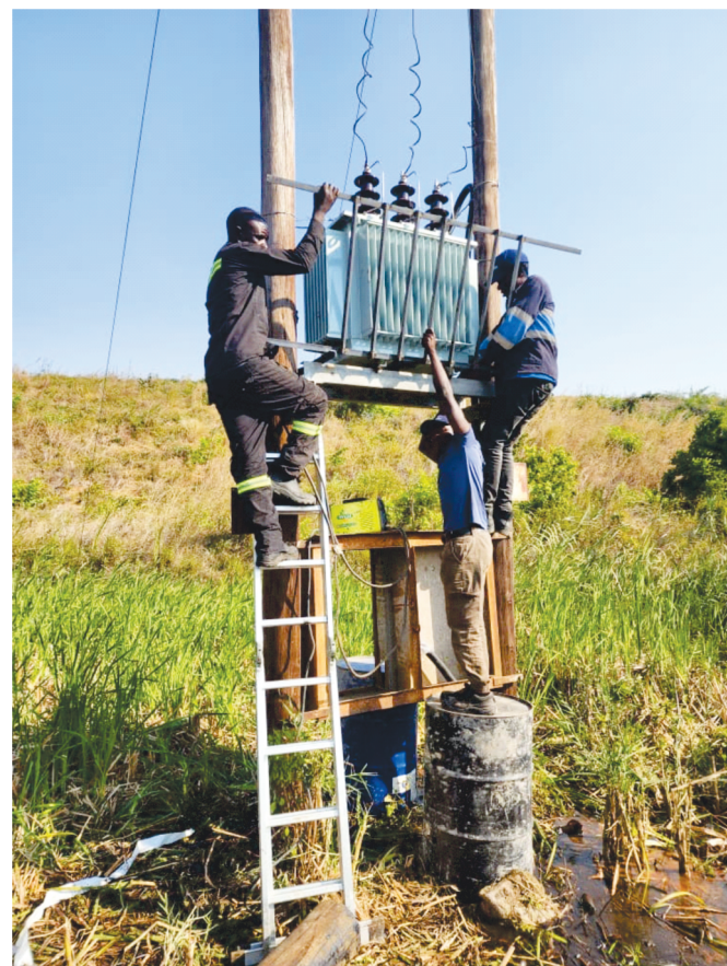
Replacement of a transformer at Chipiri Irrigation Scheme
